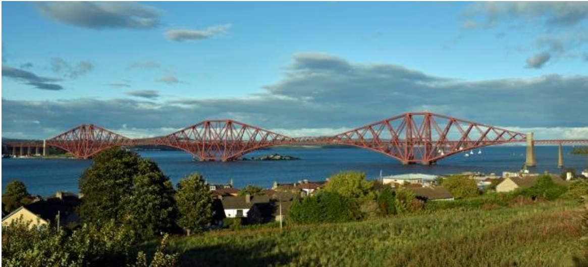
Forth Bridge in Edinburgh. Photo: Heimo Echensperger
